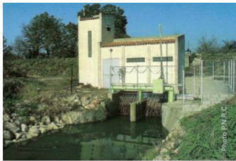
Station de pompage
